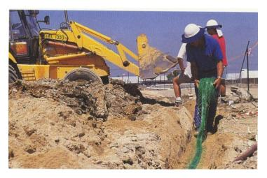
Marker tape being installed in the trench above the pipe (photograph courtesy of Iplex Pipelines
