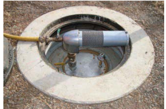
Figure 1: Vacuum test with EZIpit® test Lid assembled on the Cap and sealed with Gatic® Sealing Compound.
