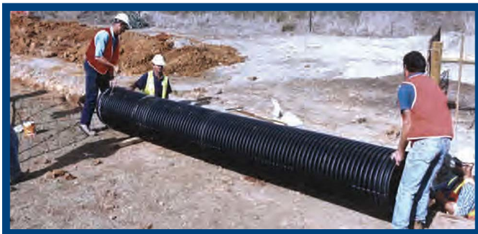
Pipes are light-weight and in most cases can be moved by hand.
