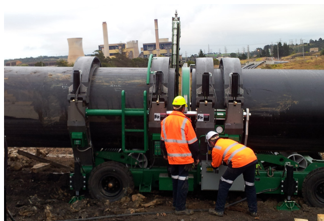
Large bore PE installation at Yallourn Power Station, VIC.
