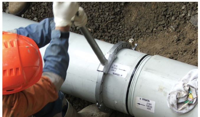
Figure 6.10 "C wrench" assembly tool used on DN300 Restrain™ Sewer Pipe
