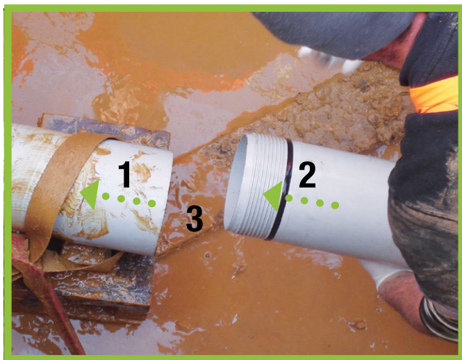
Figure 6.1 Restrain™ Sewer Pipe typical joint assembly and orientation
