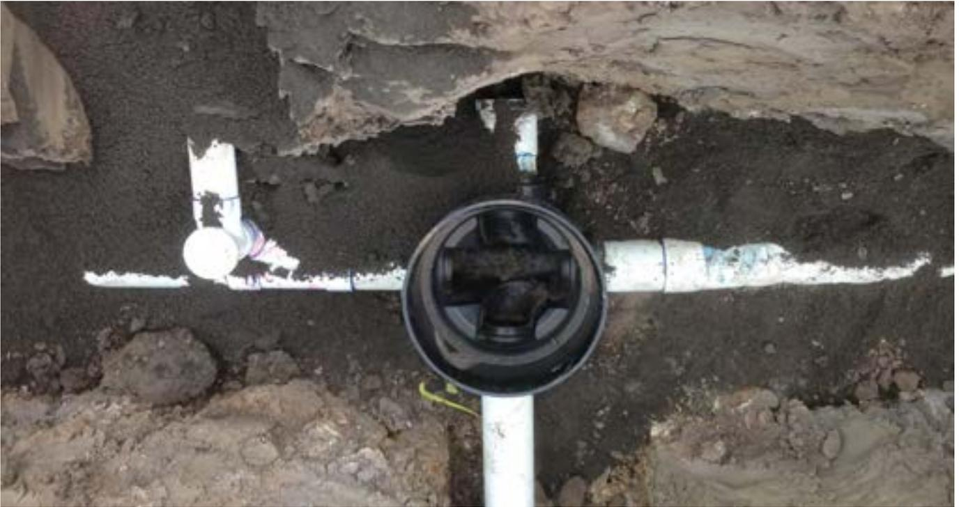
Figure 3: Iplex EZIpit® 425 MS base with 4 way 'x' profile channel and PVC DWV pipe.
