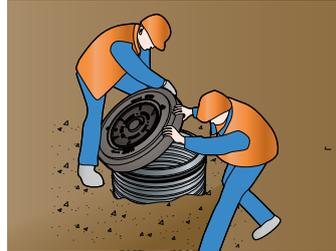
ring. Remove the lid from the cap and apply GATIC® sealing compound liberally to all vertical and horizontal seating surfaces of the lid and assemble on the cap.
