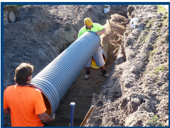
Figure 3: Pipes are light-weight and in most cases can be moved by hand.
