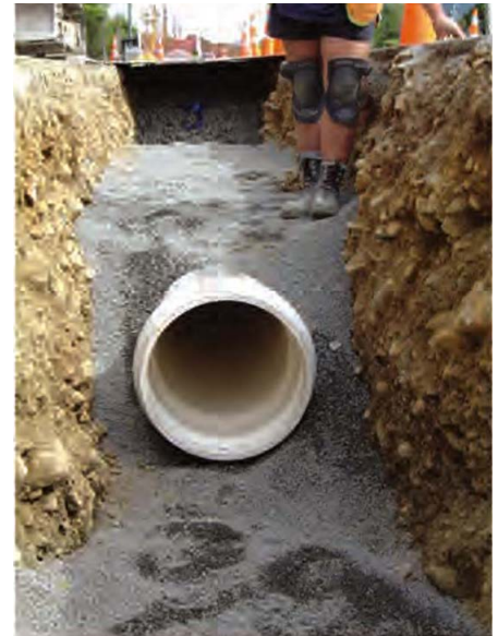
Figure 2.0 - Imported embedment material is well compacted around the pipe for support.
