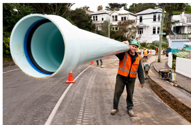
The relatively light weight nature of Iplex Apollo PVC-O pipes can allow ease of handling during installation.
