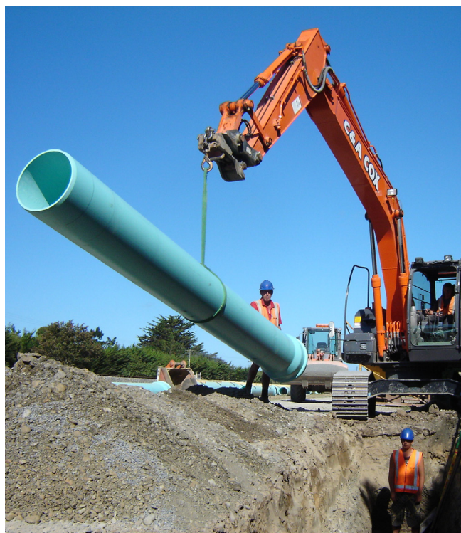
PVC-U irrigation pipe installation.
