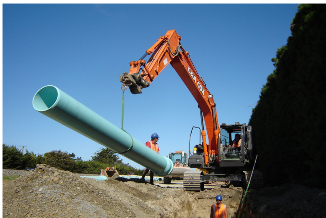
Drinking water PVC-U pipeline installed in roadway.
