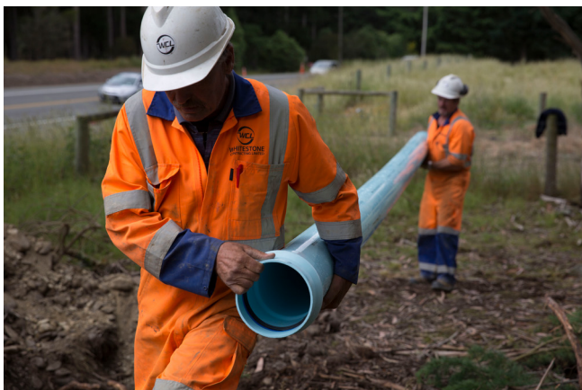
The light weight nature of PVC pipes allows ease of handling during installation.
