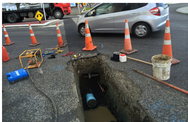
The structural stiffness of Iplex Apollo PVC-O pipe can allow installation under sealed roadways for urban pressure pipelines.
